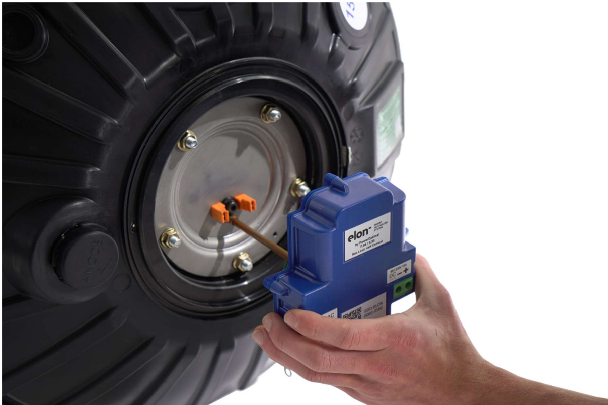
Figure 4.1. STEP 4: Insert the Elon Smart Thermostat stem at least 1/3 rd of the way into the thermostat pocket. Don't insert it fully yet.
