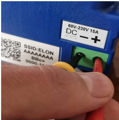
Figure A1 Checking DC voltage
